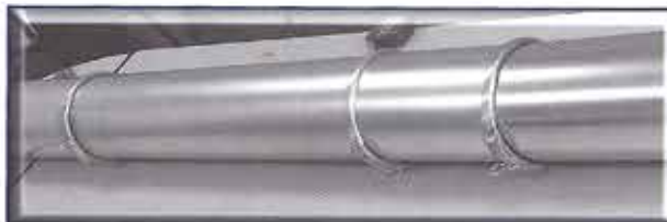
Snap clamp over O-ring and one end of nipple.
