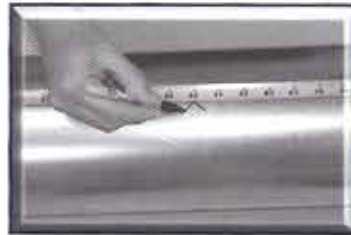
Mark distance to be spanned less 4".
