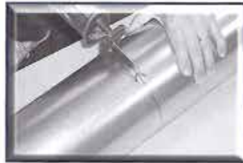
Drill access hole then cut with saw.
